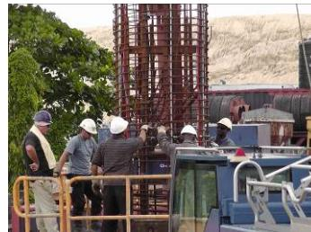
Pile reinforcing cage for TP02, with O-cell and grout pipes, being installed
