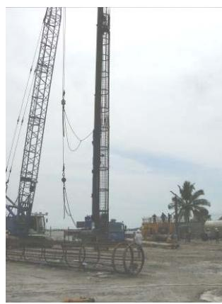
Multi-level O-cell cage ready for installation
